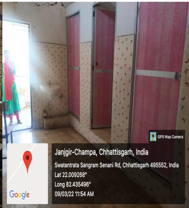
Washroom on the ground floor
